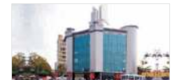
THE METRO, Rambagh Circle, Jaipur
