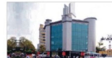
THE METRO, Rambagh Circle, Jaipur
