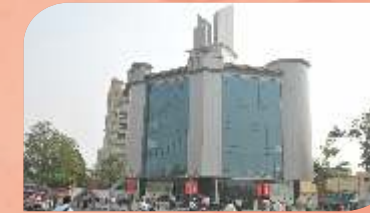
THE METRO Rambagh Circle, Jaipur
