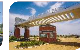
ARG INDUSTRIAL PARK Bagru, Jaipur
